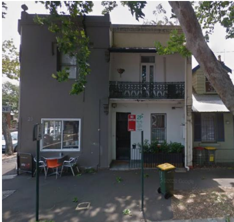
FIGURE 6: NO. 23 &amp; NO. 21 BUCKLAND STREET
