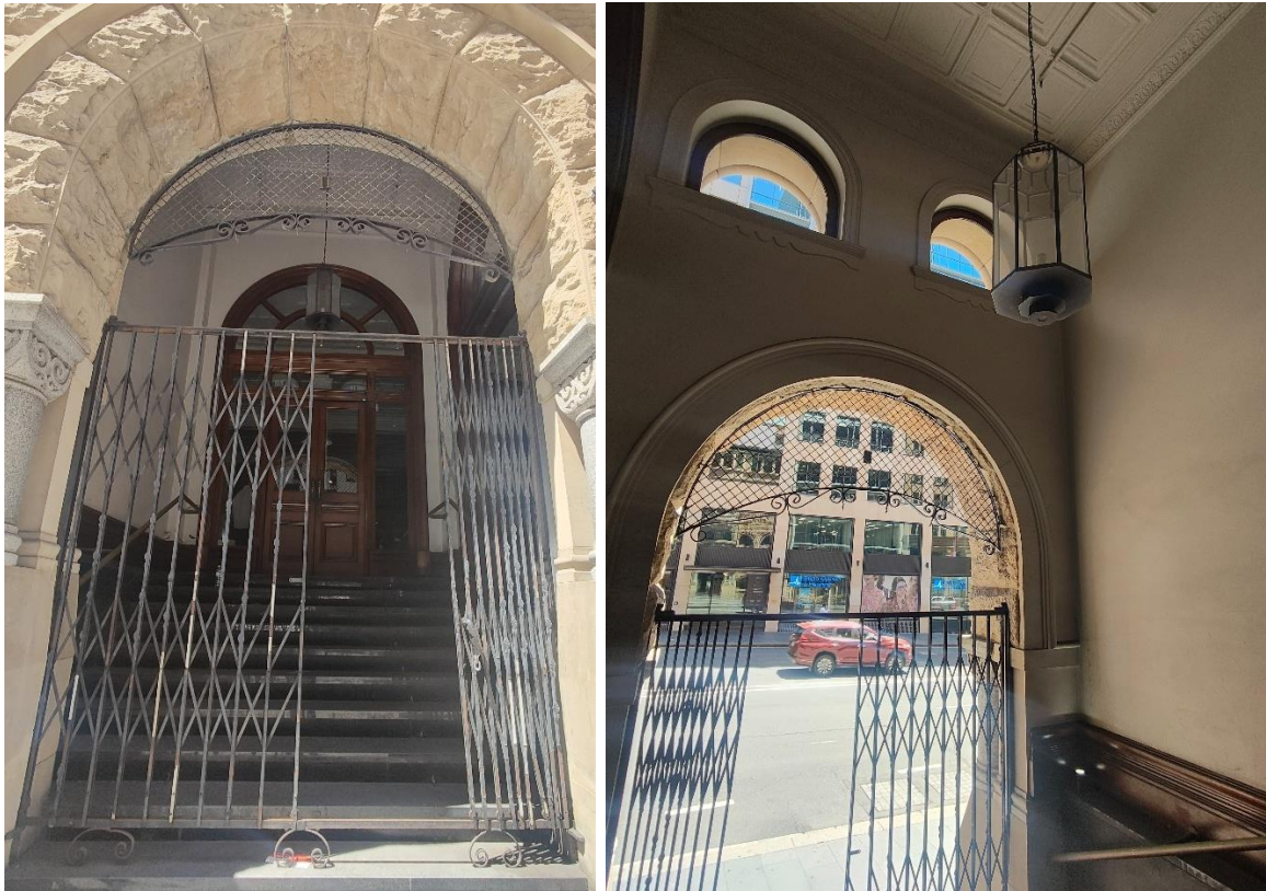
Figure 3: The step entrance of the tenancy from Bridge Street (left). The vestibule space of the entrance (right). A new neon business identification sign is being proposed on the eastern-side blank wall of the vestibule space.
