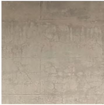
D Wall paint finish reference
