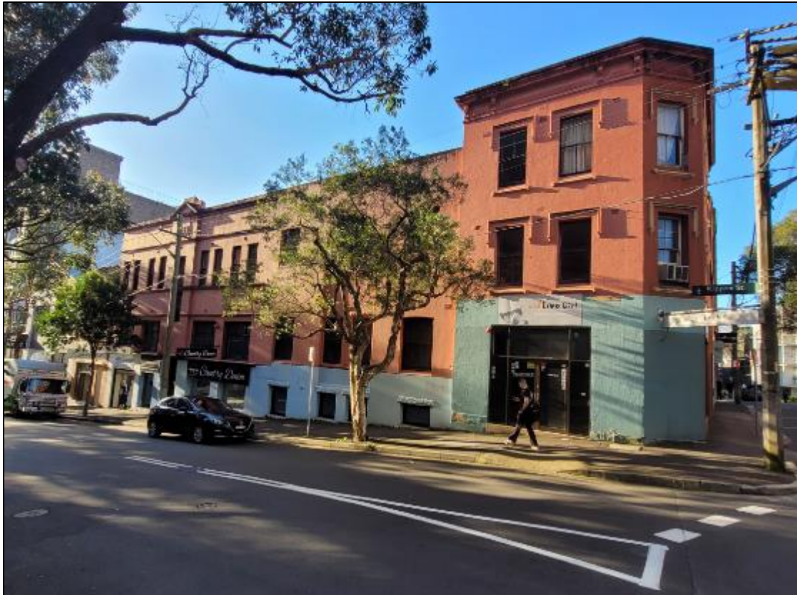
Figure 2: Site viewed from Kippax Street
