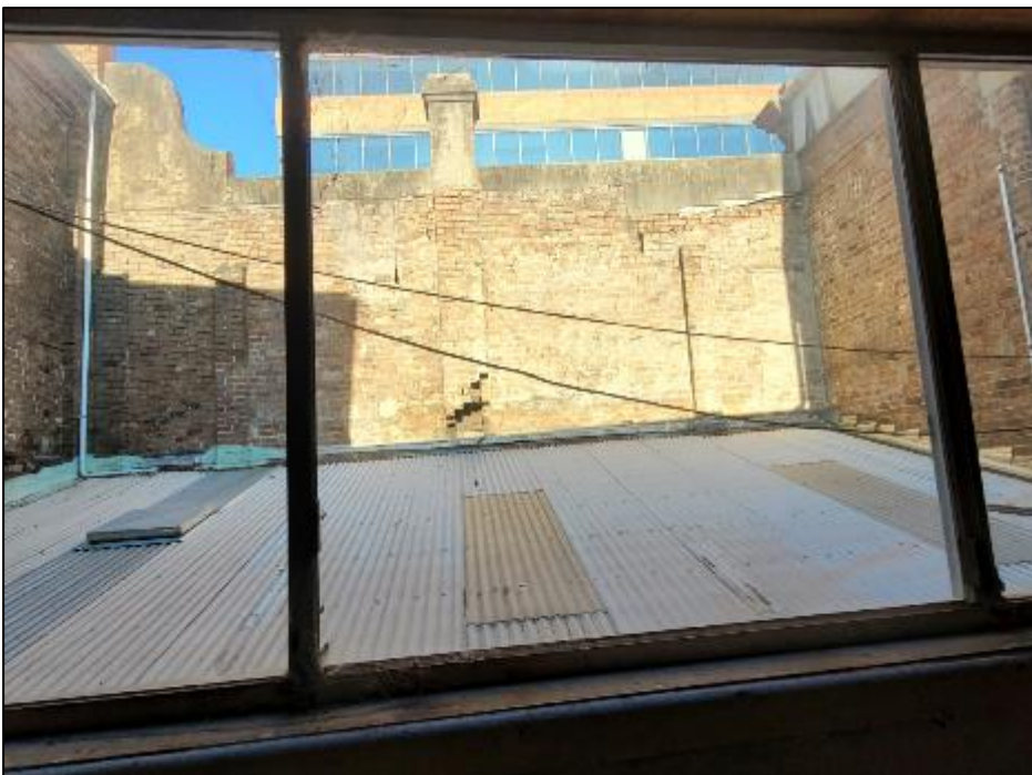
Figure 9: View of the parapet of the looking south-east towards Waterloo Street
