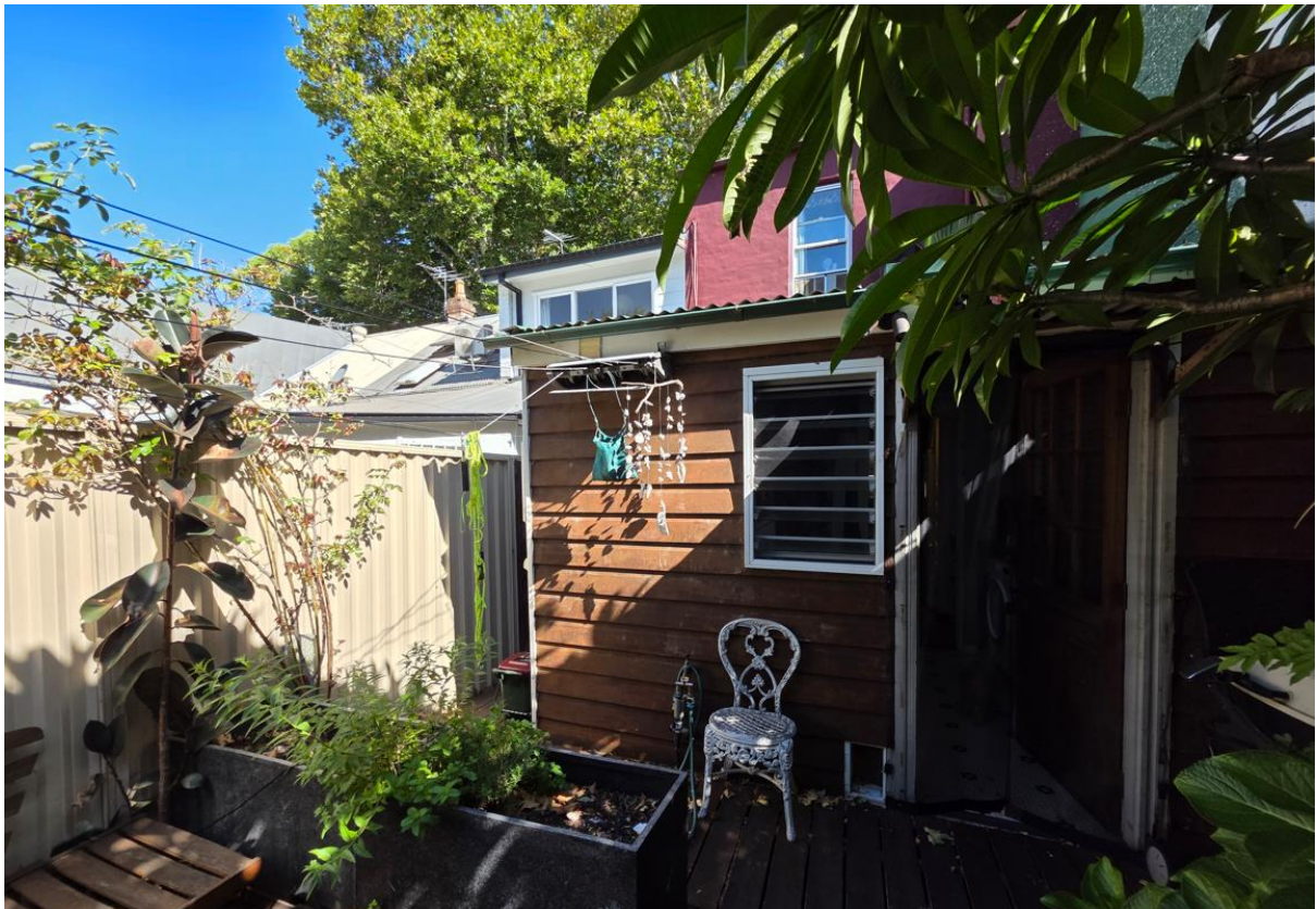
Figure 6: South-facing view of rear yard and building
