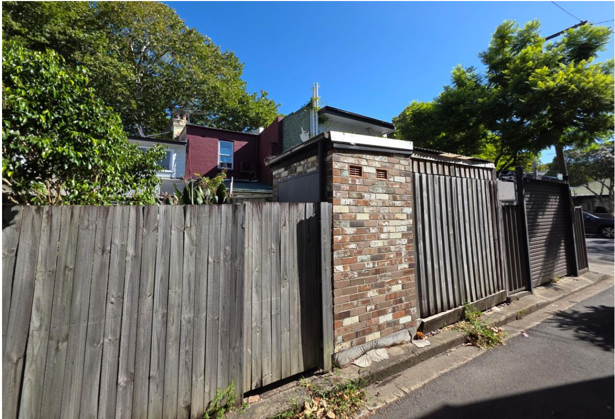
Figure 3: Rear of site (maroon building and shed at rear) viewed from Wyndham Lane facing south
